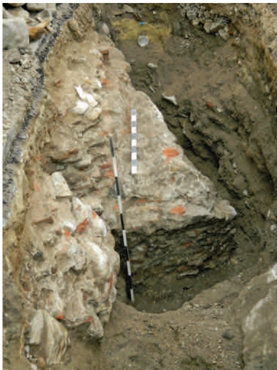
Fig. 6. Structure of the Tower Gate foundation.
