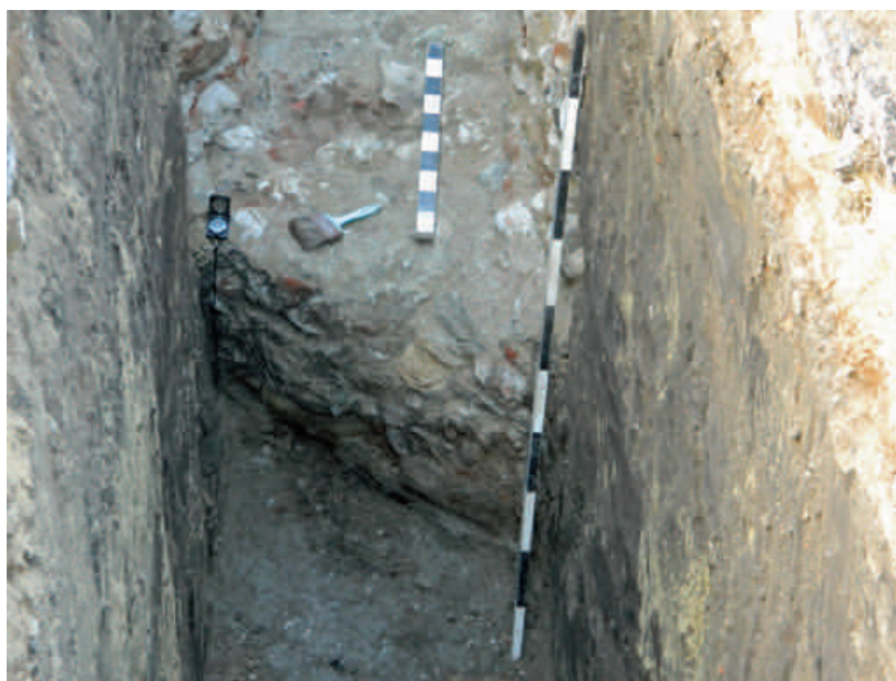
Fig. 15 Detail of the foundation.
