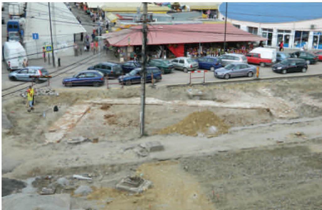
Fig. 29. General image of a part of the walls of the Tower Gate Bastion.
